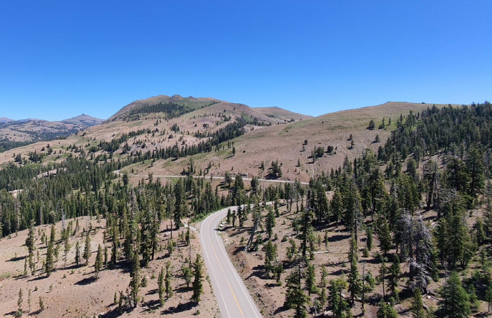
Paved Road in Alpine County
