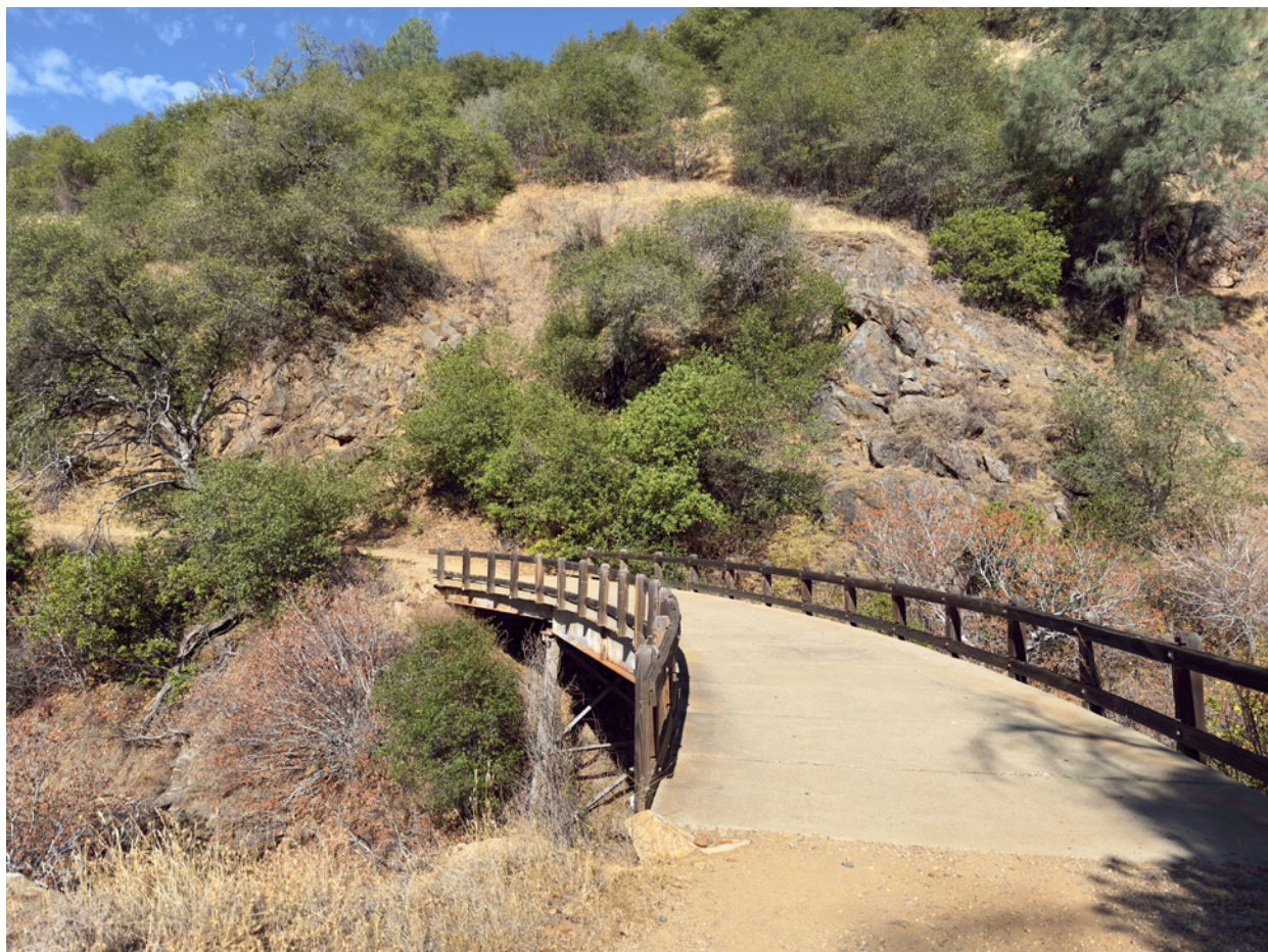
Soft Surface Road near El Portal
